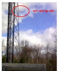
The club recently purchased a Telewave ANT 160D VHF antenna which was just installed on the new South Killingly (SK) tower at the 130ft level. This
